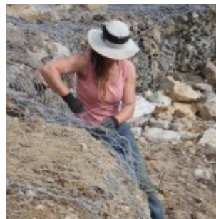
Lisa repairing the spillway on our dam
